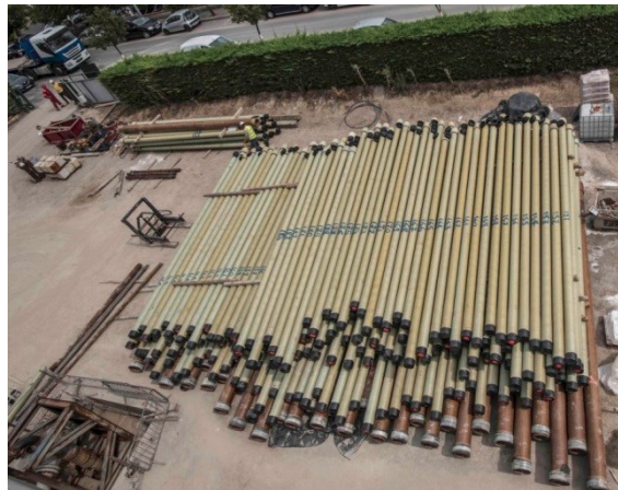
Figure 12: Composite casing on the platform in Bonneuil (GPC IP)
