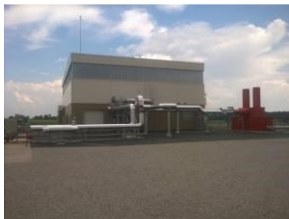
Figure 14: The Rittershoffen geothermal heat plant (source: ECOGI)
